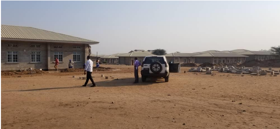
Figure 11: Chikwawa TTC under Construction
