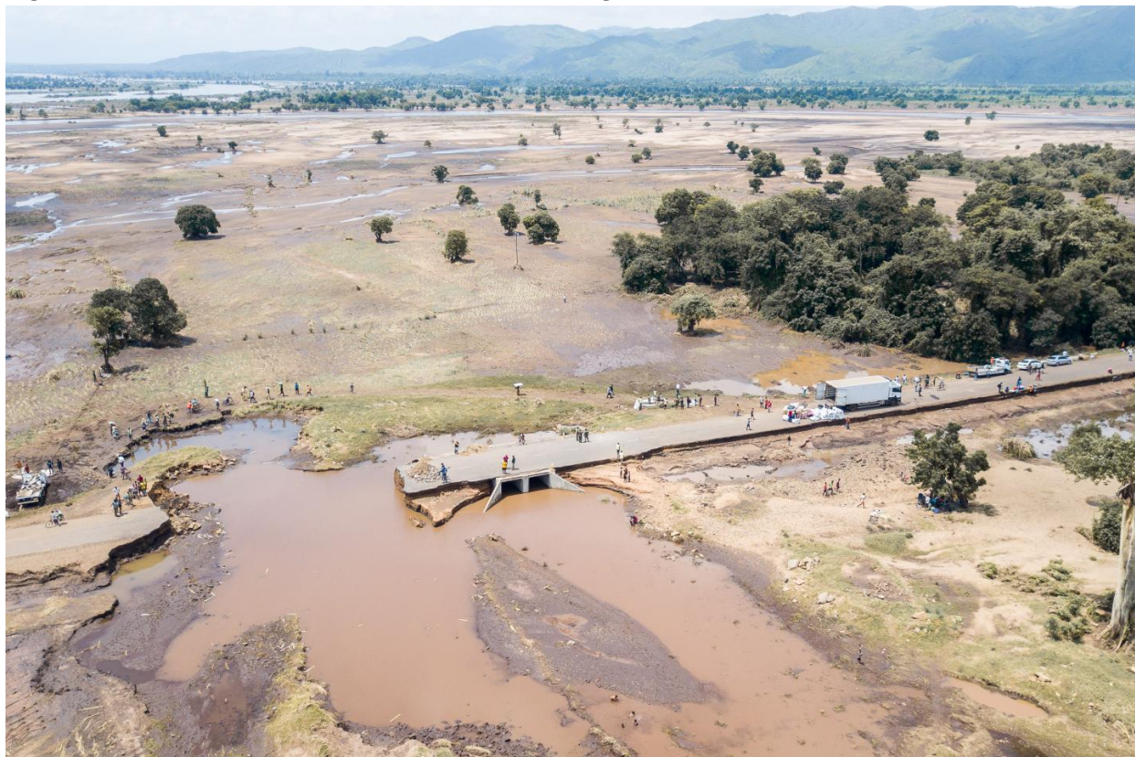
Figure 17: M1 Road cut off by 2022 Flooding at Chikwawa Boma
