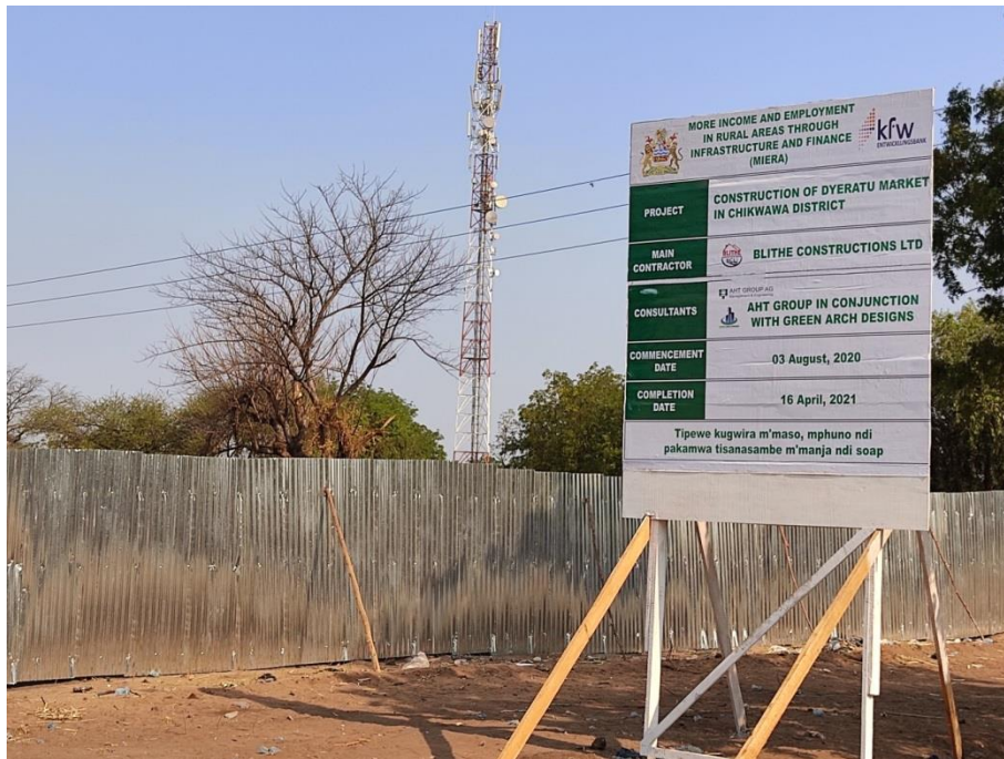
Figure 5: Dyeratu Market Construction Site
